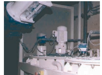
Duwa-Matic® 650 installation integrated below the existing silo
