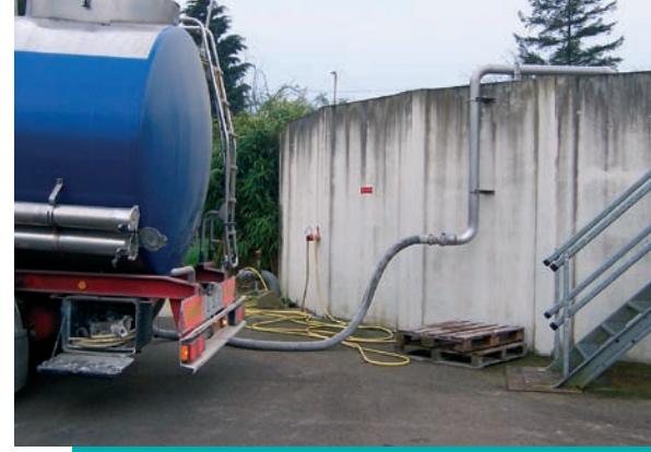
Tanker delivery of liquid Neutralac® SL30 to the sludge storage tank
